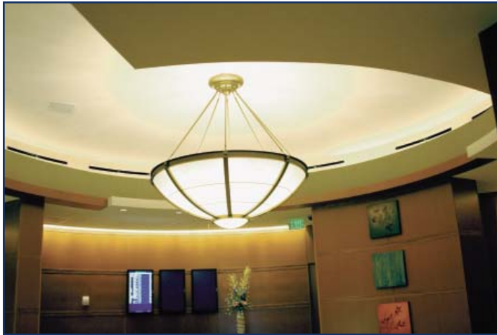
Figure 3: Curved FlowBar diffusers in the entry from the terminal into the Grand Hyatt hotel reception area.
